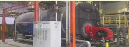
Fuel-Fired Boiler
